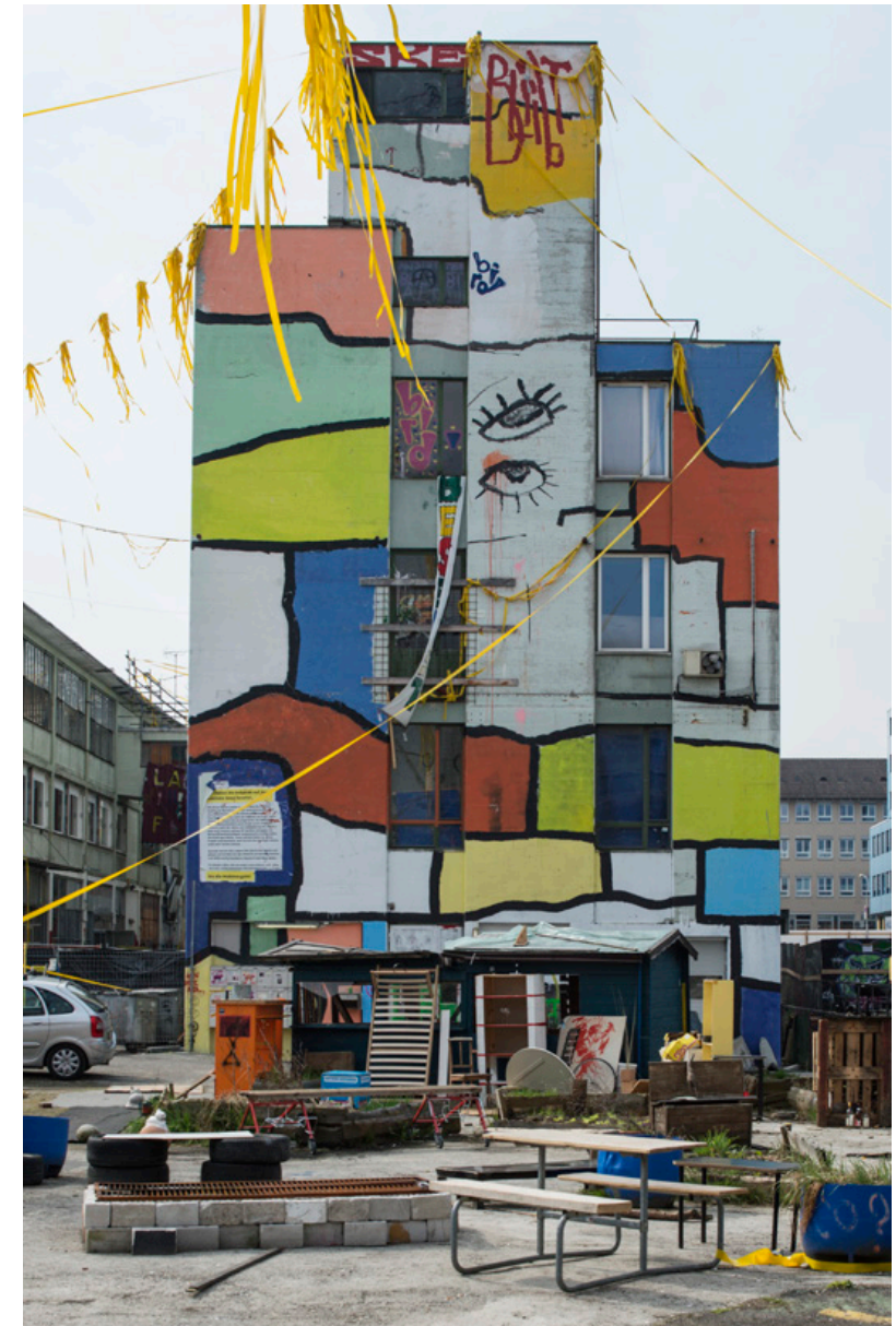
2014: The occupied Labitzke site in the Altstetten quarter of Zurich.
