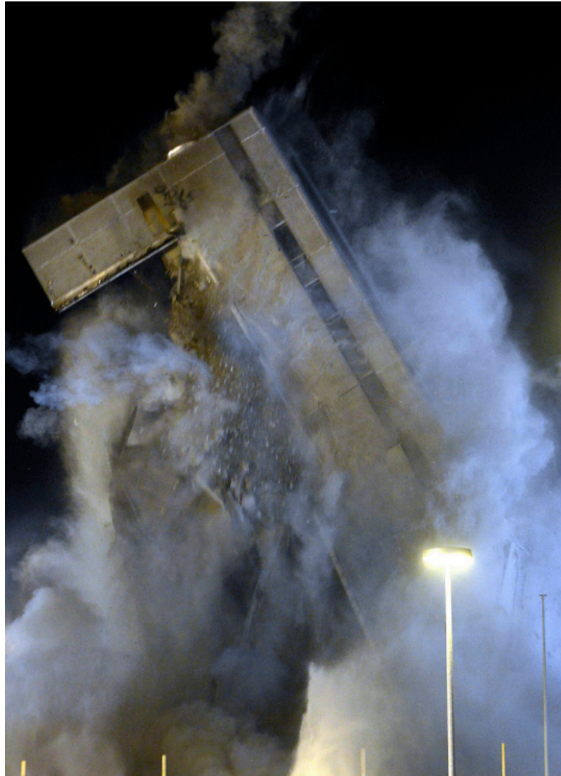
March 2013: The Sprecherhof building in Aarau is demolished.
