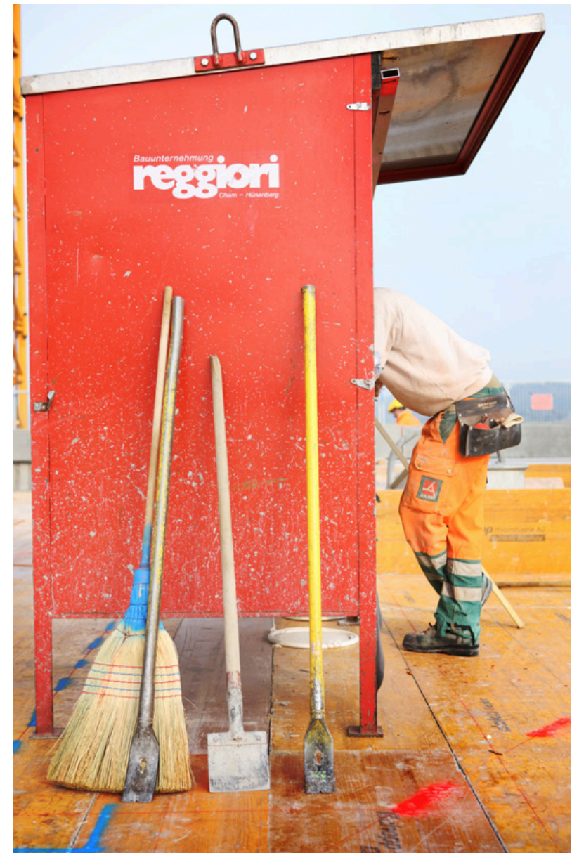
April 2010: Construction work on Mobimo Tower.
